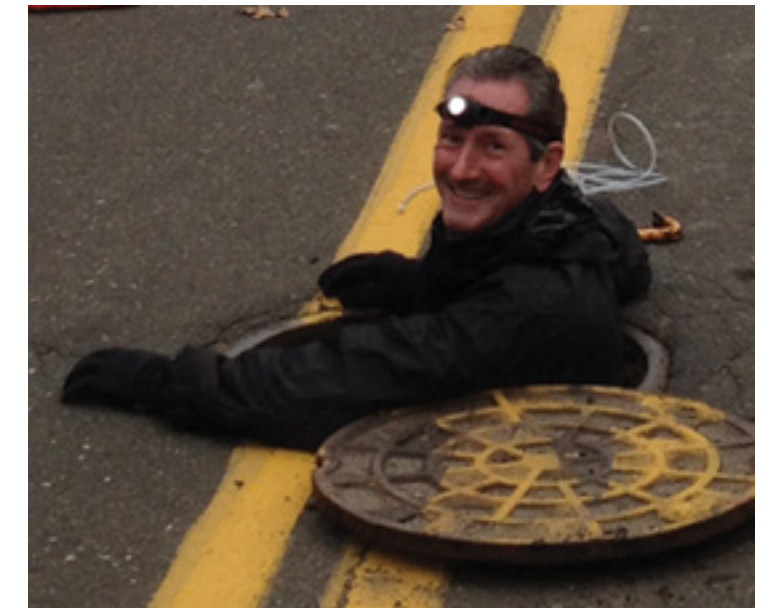
Gaboury Benoit has taken a very hands-on approach to monitoring how well a network of bioswales across New Haven are performing — even descending into the city’s stormwater drainage system.
